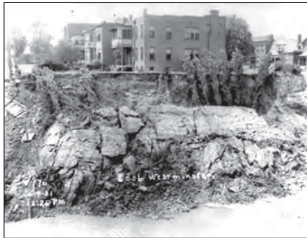
River DesPeres collapse 1931.
