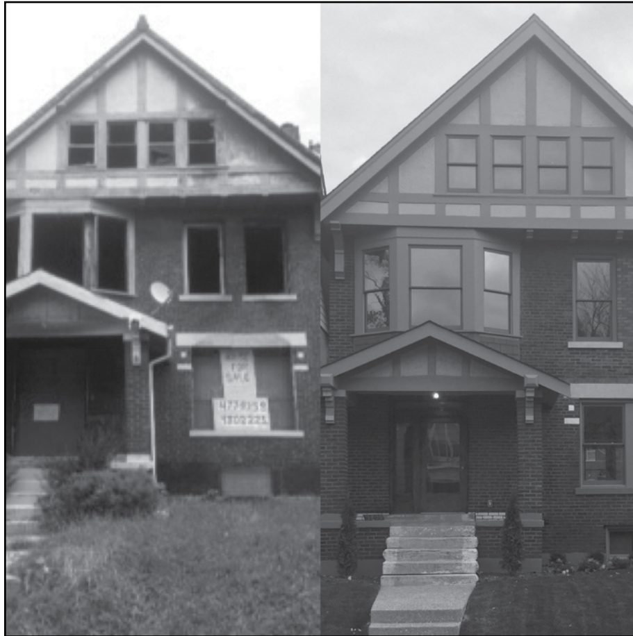
Before and After shots of 5859 DeGiverville, rehabbed by Eric Trudo after a devastating fire left the building empty and abandoned.
